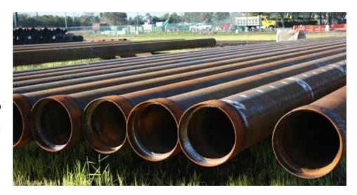
"Due to the varied geology of the region, steel pipe piles proved superior to prestressed concrete piles, as they could be stored on-site and spliced to create the longer pile lengths needed for this project"
